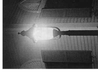
Decorative streetlights should avoid glaring fixtures such as the one shown on the above left. The better design on the right positions the bulb near the top of the fixture. Light is sent downward where it is needed rather than wasted.
